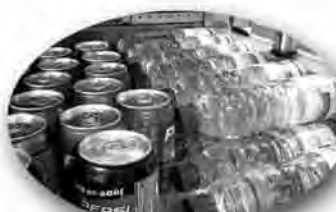
K. Multiple stacking restricting cold air movement in the deck/ base
